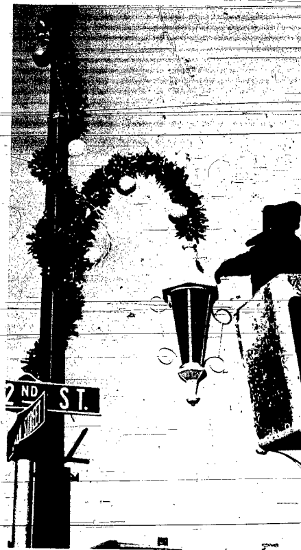
CHRISTMAS LIGHTS were being installed on Main Street Monday and Tuesday in Wayne. A crewman from Norfolk makes a final inspection of the decorations he has just placed on a light pole Tuesday afternoon at Second and Main Streets. Roger Elder, manager of the Wayne Chamber of Commerce, says the colorful panorama of new holiday lights will be turned on Nov. 28.
